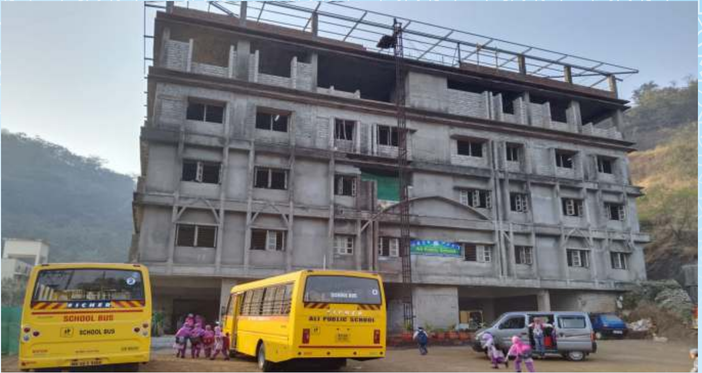
Front View of the Building
