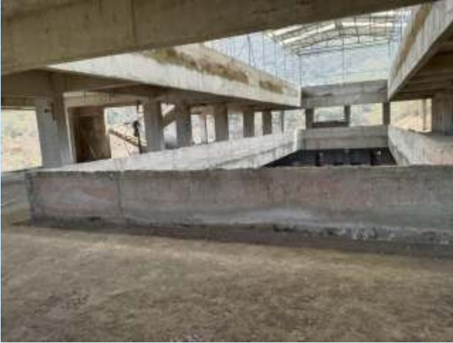
School Building Top Floor
