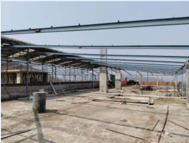
School Building Rooftop
